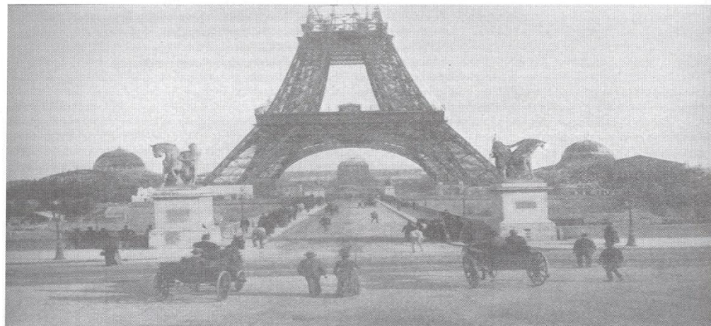
Playing near the half-built Eiffel Tower.
